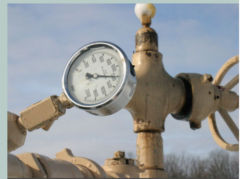
A gauge fitted on a CO 2 injection pipe measures pressure during an enhanced oil recovery effort.
